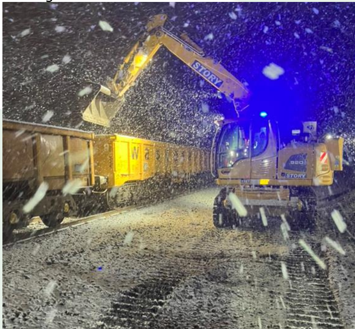
Night works underway between Holywell and Seghill during the recent snow
